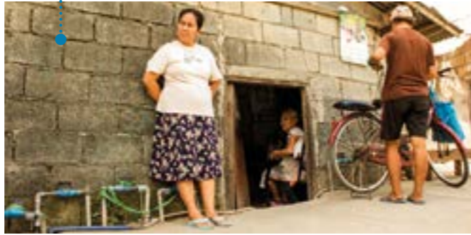
Floods deposited silt and mud in front of this house in the Philippines. For an elderly person with mobility aids it is difficult to enter and leave the house.
