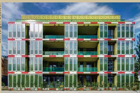
The BIQ House in Hamburg generates energy from the algae biomass in its façade.
